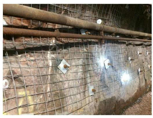
Figure 2.4. Veined and sheared amphibolite that corresponds to a zone of decreased seismic velocity between the East and West Access Drifts near Drill Stations 1 & 2.
